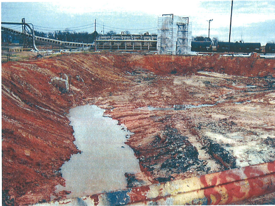
Photo 1. Excavated pond January 8, 2014.
